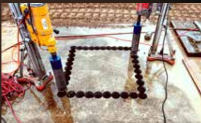
CONCRETE OPENING (BY STITCH CORING)
