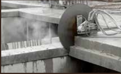
CONCRETE CHAMBER CUTTING
