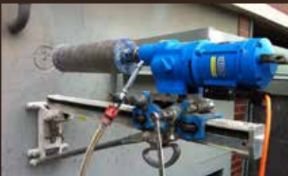
CONCRETE BEAM CORNING
