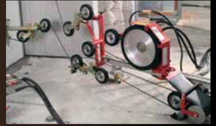
COLUMN DIAMOND CUTTING
