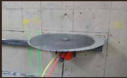
CONCRETE WALL CUTTING
