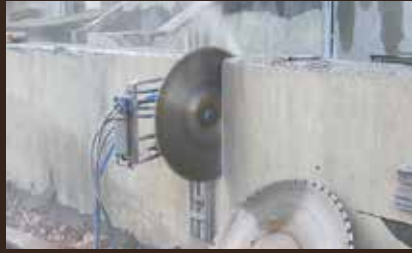
CONCRETE COLUMN CUTTING
