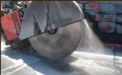
CONCRETE FLOOR CUTTING
